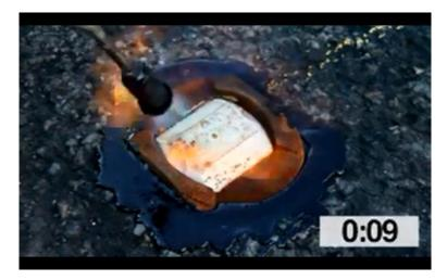
2. Chisel the old/worn reflector from the casting, you may still need to apply heat to do this
