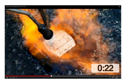
3. Completely remove the old/worn reflector casing scrapping any excess glue from the base of the casting until clean
